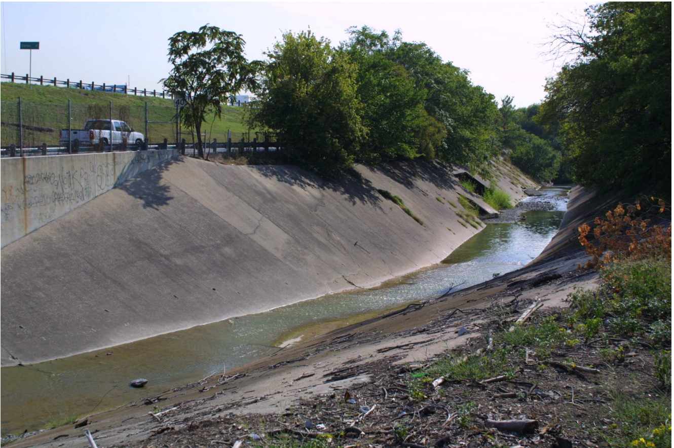
Streambed paved during Fort Worth Turnpike construction in the mid-1950's —August 2003
