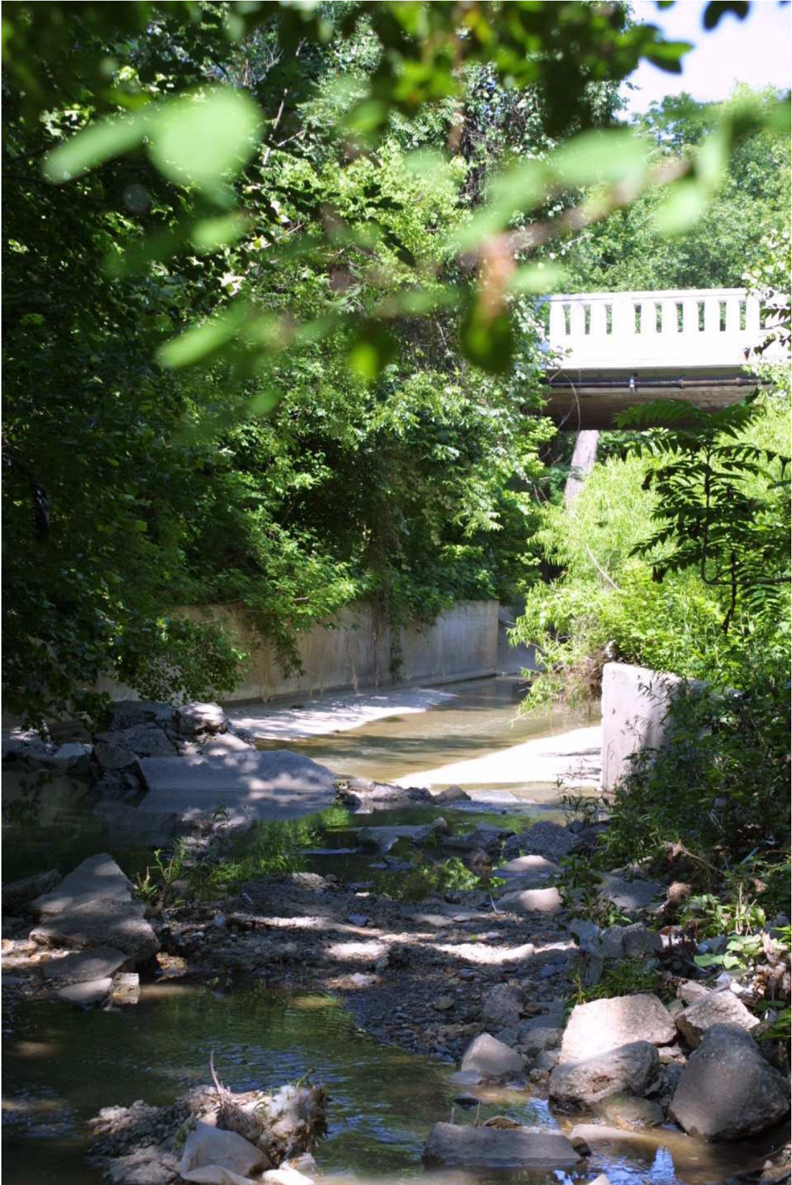
Total concrete creek bed lining south of the Edgefield Street bridge—May 2003
