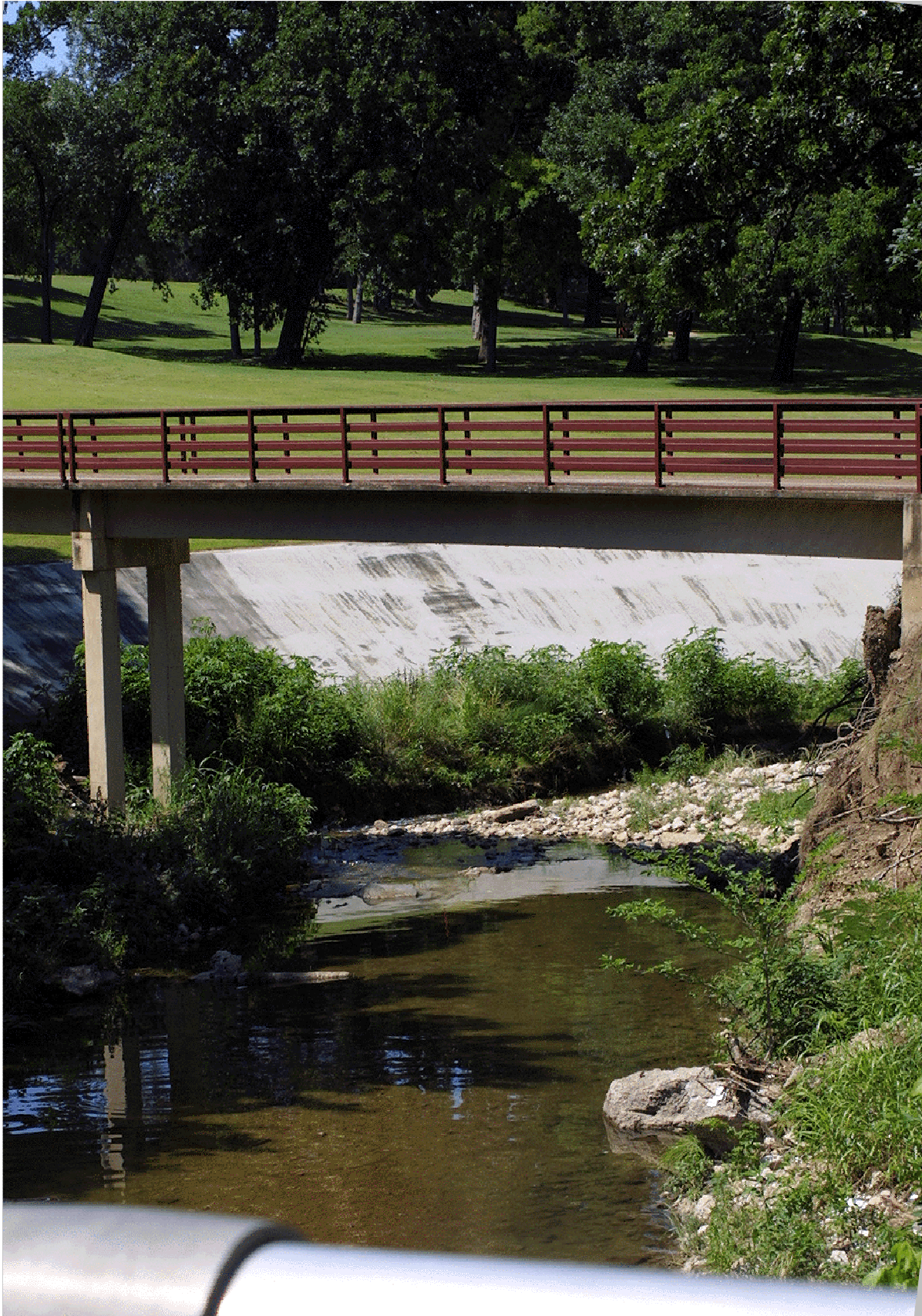
Concrete paving of west creek bank, north of the Colorado bridge—May 2003
