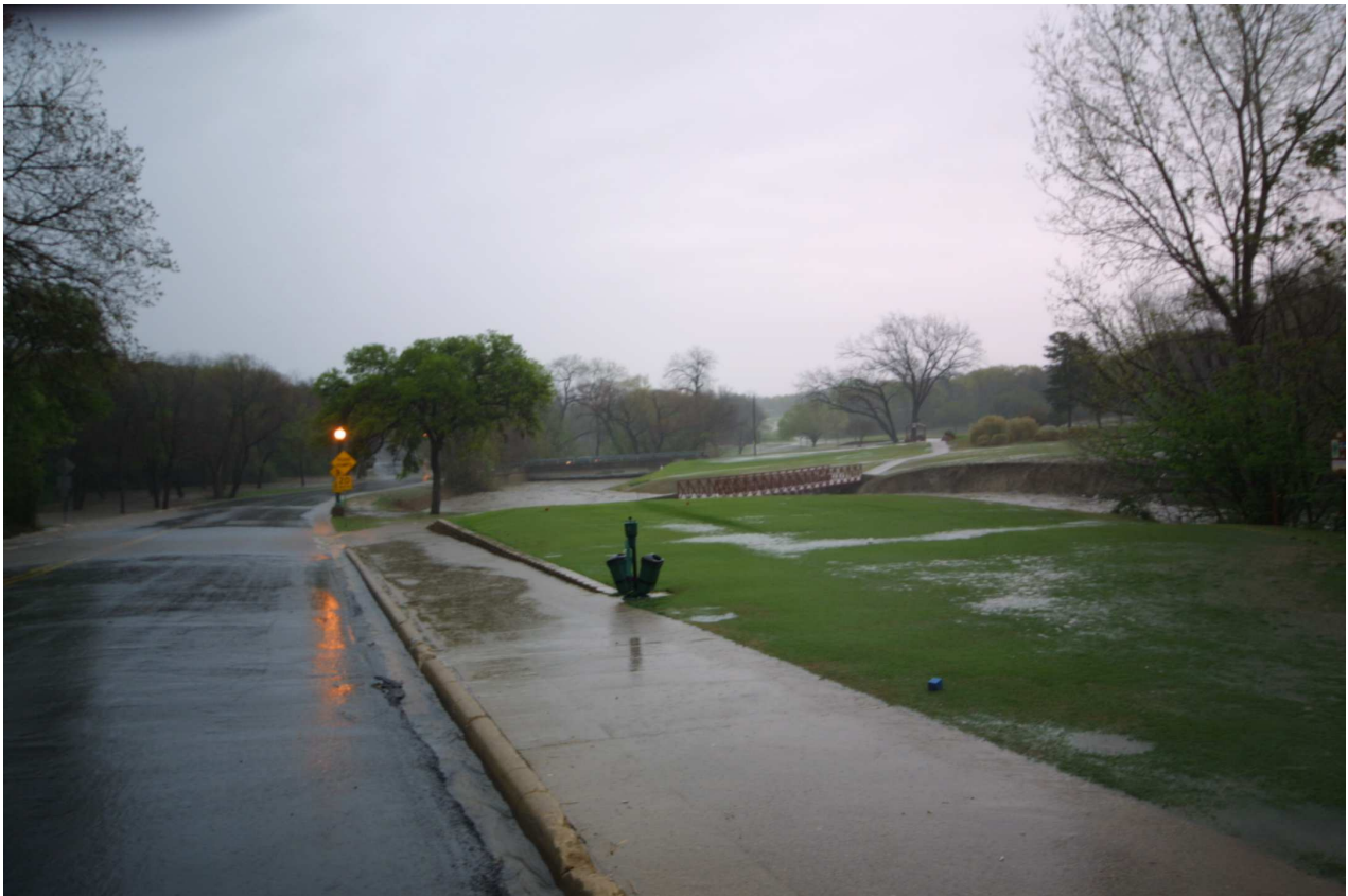
Coombes Creek floodwaters at the North Oak Cliff Boulevard bridge—about 1:45 p.m. on Sunday afternoon the 19 th of March 2006. Rushing water almost completely fills the bridge's opening for runoff flow.
