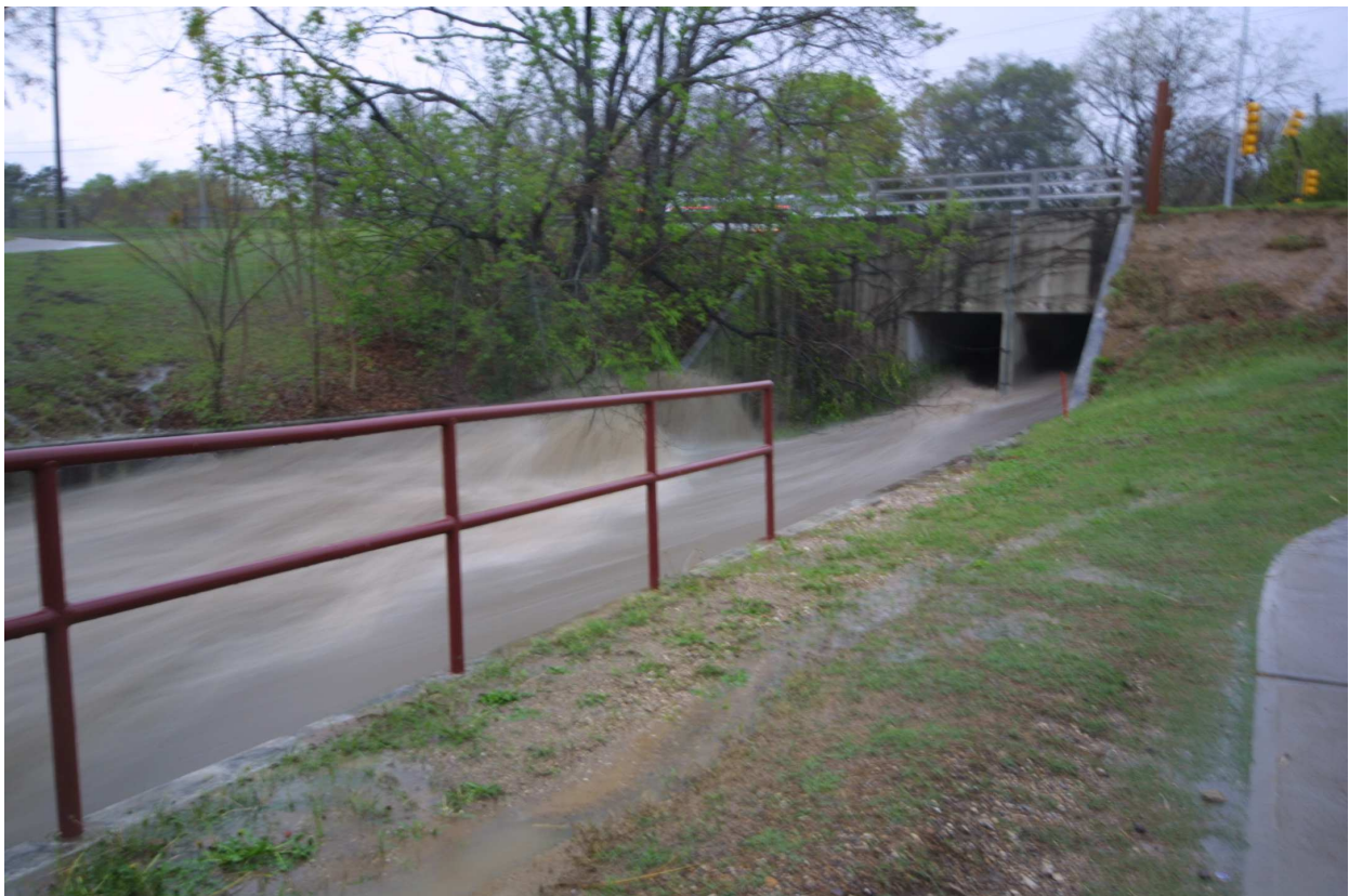
Coombes Creek floodwater runoff at Hampton Road bridge—about 1:45 p.m. on Sunday afternoon the 19 th of March 2006. Water rushes under the bridge at what seems like forty or fifty miles an hour, making a constant frightful roar.
