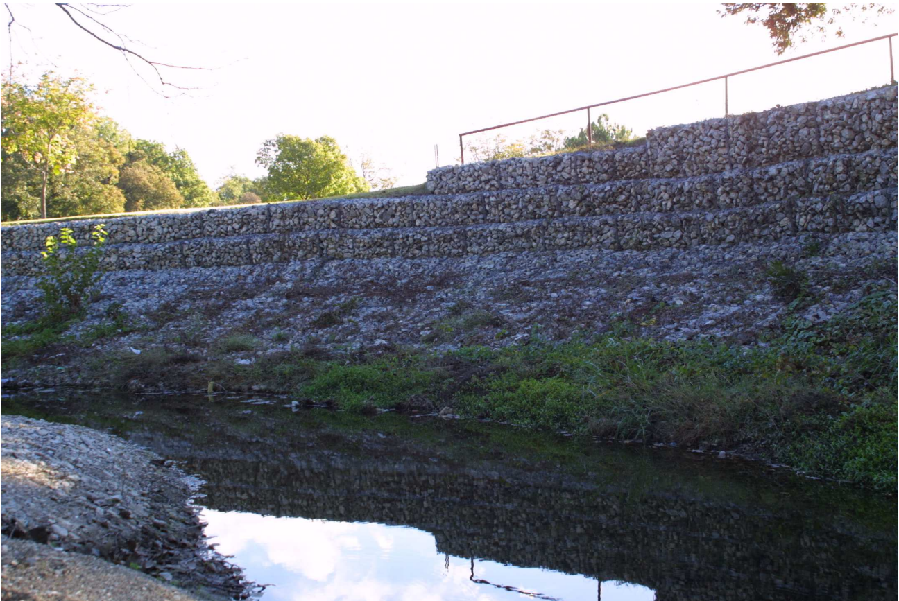
Small loose Austin limestone held in place with galvanized wire basketry-- downstream from N. Oak Cliff Blvd. bridge --- October 2003
