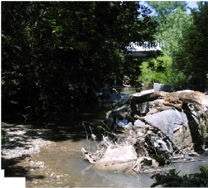
Composite photo showing mass of toppled masonry from a former erosion control attempt and giant teetering tree, just upstream from the Edgefield bridge—May 2003
